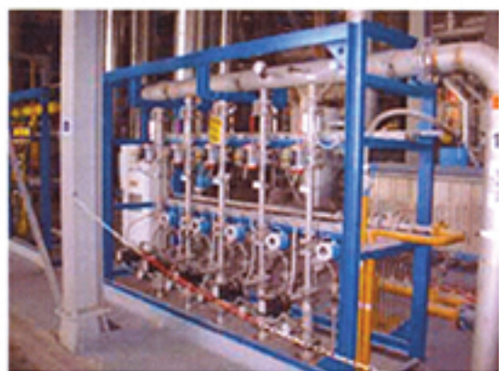
Figure 3: Air Liquide Altac NCE valve train.
